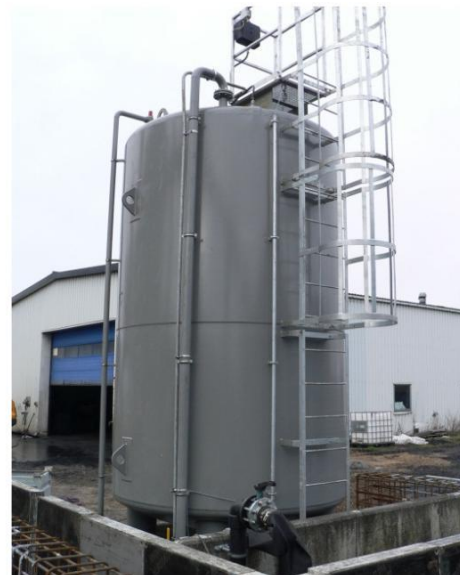
20 m 3 tank diameter på 2500 mm. With ladder and platform on top of tank, fill point to ground level, leak detection system etc.
